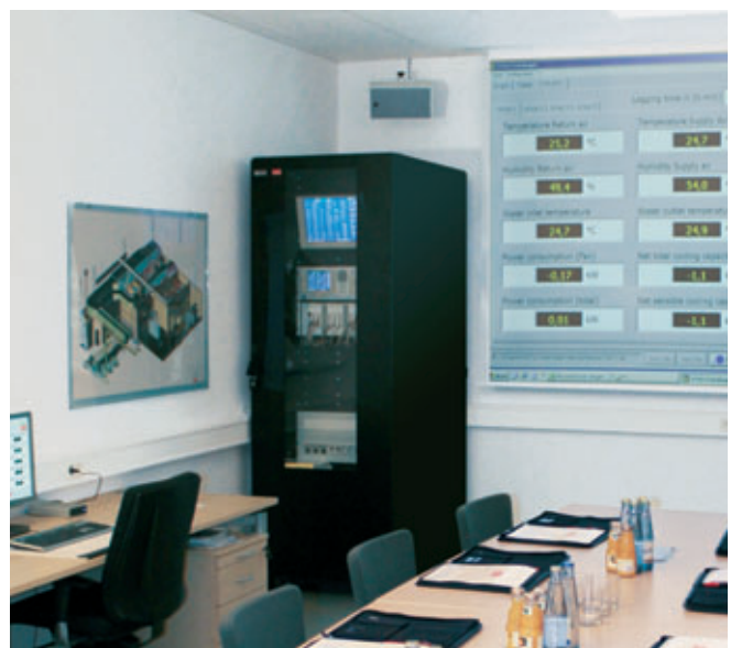
Experience the testing of your air-conditioning system live in our control room
