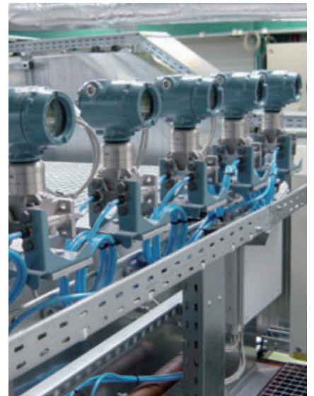
Pressure sensors for conditioning system
